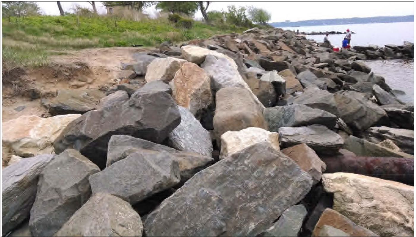
Riprap shoreline near the intake, facing south 2
