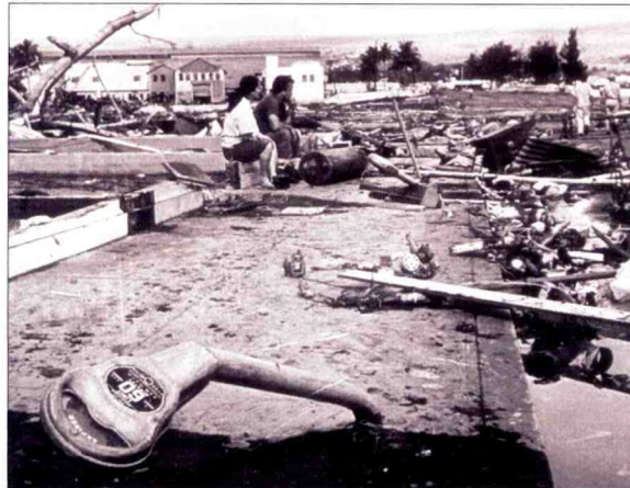
Figure 1. Tsunami damage in Hilo, Hawaii, 10,000 km from the 1960 Chilean earthquake. Hilo suffered 61 deaths and $24 million (not adjusted for inflation) in damage.
