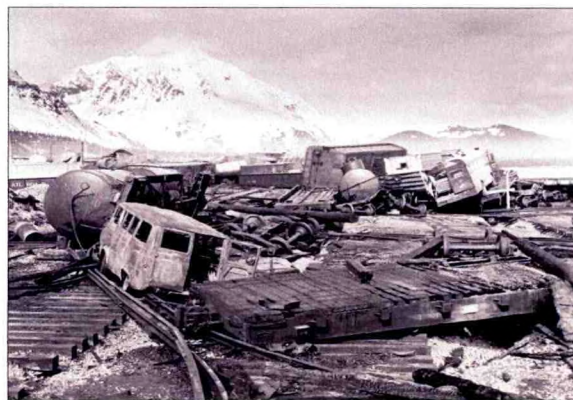
Figure 28. March 28, 1964 Prince William Sound, Alaska. Tsunami damage at Seward, Alaska.
