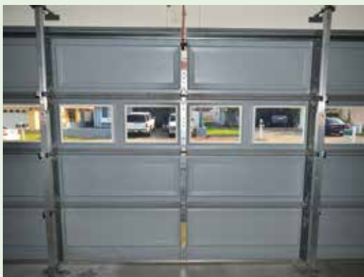
Figure 5-23. Vertical braces such as these can be deployed during high-wind events to strengthen the garage door. The braces are secured from the header over the garage door to the fasteners installed in the concrete floor. Deployment and breakdown are about 10 minutes each. The windows have been covered with a laminate film. Image courtesy of Dennis Hwang
