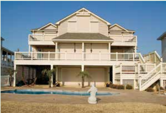
Figure 5-11. Coastal home protected with roll-down shutters on all windows and doors. The shutter is held in place by vertical guide tracks and can be deployed manually or with an integrated electric motor. Image courtesy of QMI Inc.
