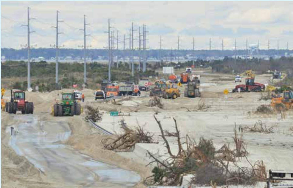
Figure 2-4. Following Superstorm Sandy in October 2012, more than 40,000 tons of sand that the storm had deposited from storm surge and flooding had to be removed from Route 1 to reopen the vital road through coastal Sussex County. Photo by Ron MacArthur
