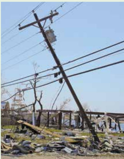
Figure 5-25. Downed or damaged power lines in a residential area can pose a serious danger to public safety. Image courtesy of U.S. EPA
