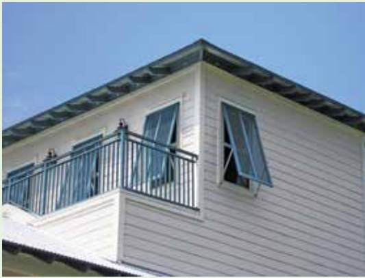
Figure 5-13. Bahama shutters made from durable extruded aluminum components add “islands” flair to a home and provide effective opening protection. Image courtesy of Roll-a-way
