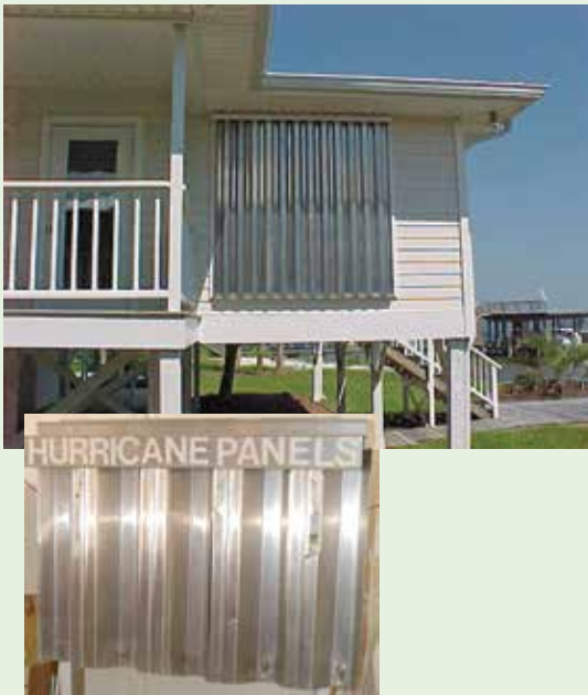
Figure 5-14. These 0.050 gauge aluminum storm panels offer cost-effective storm protection. In this example, panels slip into a track above the window and secure onto a bottom track using wing nuts. Image courtesy of Roll-a-way
