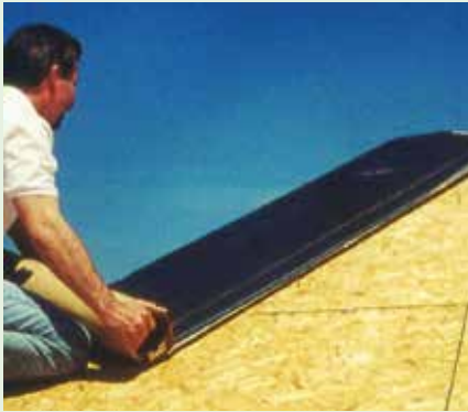
Figure 5-10. Synthetic underlayments are typically made from polypropylene, polyester, or fiberglass fabric, which weighs less than felt building paper, can be manufactured with anti-slip surfaces, and can withstand exposure to the elements for six months. Image courtesy of Carlisle Coatings & Waterproofing
