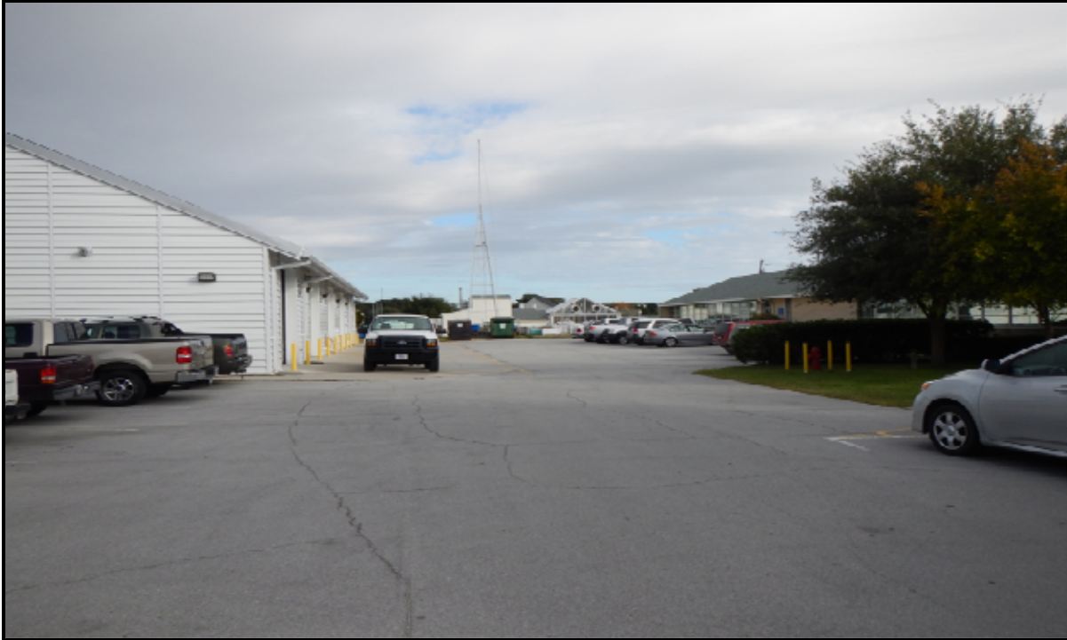
Photograph 9: View of the northern parking lot and location of the proposed location of the underground utility conduit facing east.
