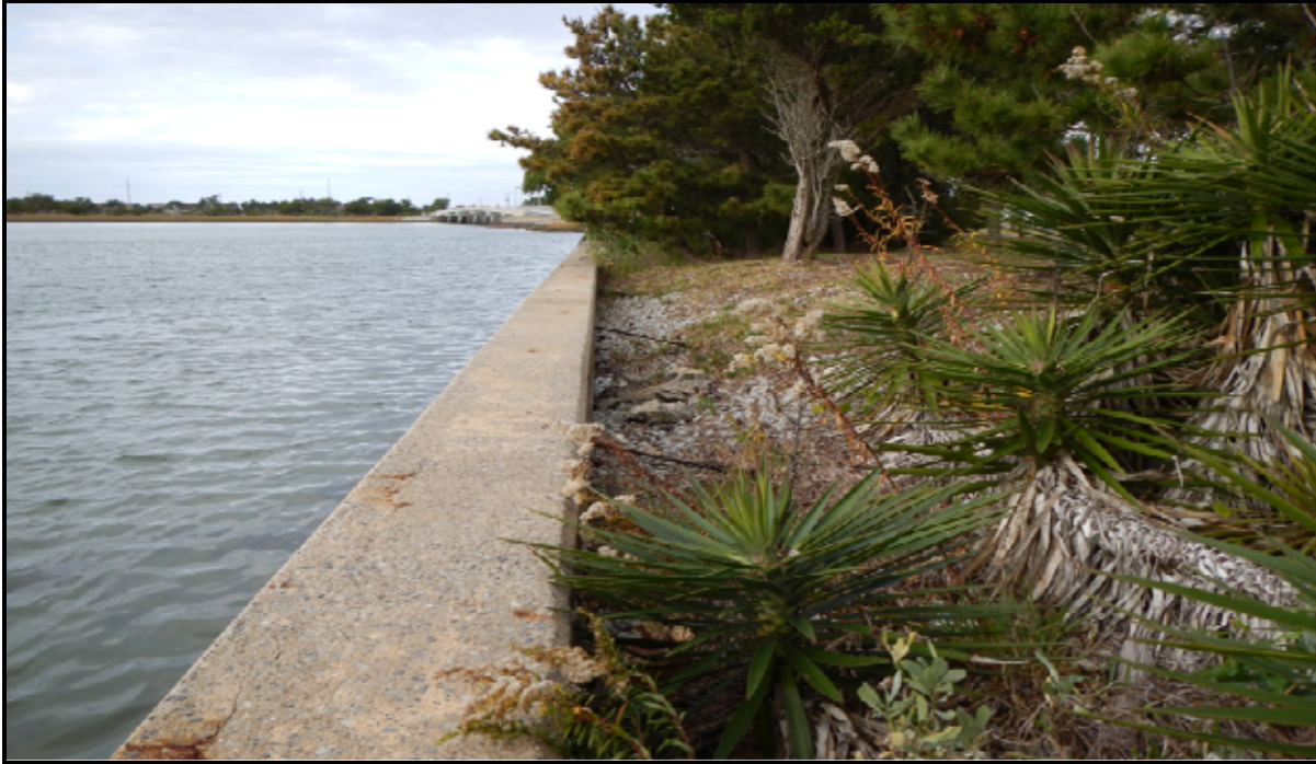
Photograph 13: View of the exposed stabilization rebar installed on the existing seawall.
