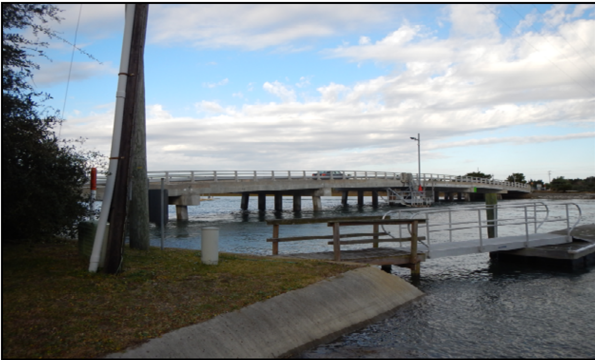
Photograph 14: View of the northern access bridge and the platform containing the hose reel that is proposed to be moved to accommodate the electrical conduit on the side of the bridge.
