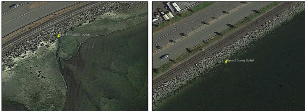
Figure 4. Riprap lines the shoreline surrounding the existing outfalls (adapted from Figure A-6 of Appendix A in the Biological Assessment).
