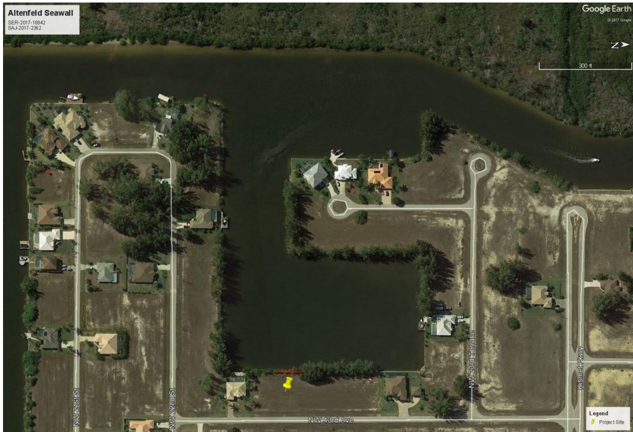
Figure 2. The project site at 2216 NW 43 rd Avenue, Cape Coral, Lee County, Florida. The red line indicates the 85 linear feet (lin ft) of unconsolidated shoreline under consideration in this project (©2017 Google).
