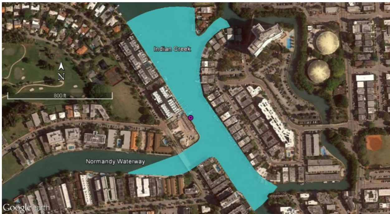
Figure 3. Image depicting the Normandy Ventures, LLC, action area (light blue); the existing docking area is above the purple dot (background image ©2017 Google Earth)
