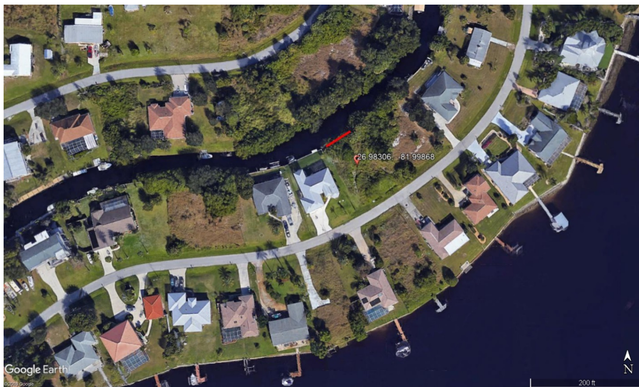
Figure 2. The project site at 3203 Peace River Drive, Punta Gorda, Charlotte County, Florida, in a tidal manmade canal showing 70 lin ft of unconsolidated shoreline (©2017 Google).
