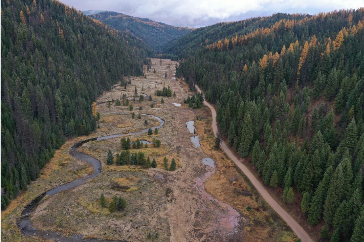
Figure 3. Looking downstream at the Crooked River post construction (2017–2021). Project construction includes developing wetlands in low areas along the left bank of Crooked River. Some of these low areas have been connected to the main channel via side channels to provide more off channel habitat.
