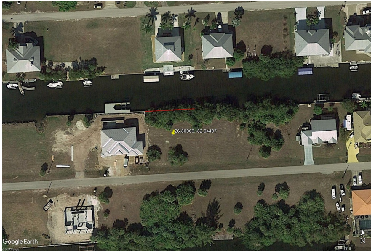
Figure 3. Imagine showing the existing undeveloped, residential property and unconsolidated shoreline at 24310 Blackbeard Boulevard in Punta Gorda, Charlotte County, Florida. The red line is the approximate location of the new seawall (©2017 Google).
