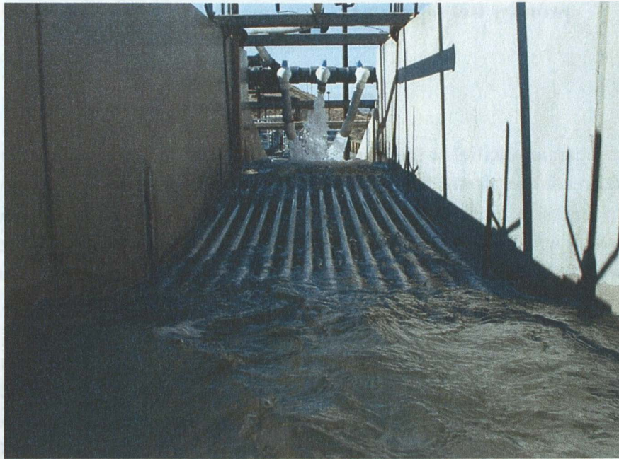
Figure 3. Large fish separator in high-velocity flume test facility at Ice Harbor Dam, 2000. The camera view is from inside the flume looking downstream, showing water surface elevation change at the separation bar/adjustable slope flume interface. Note the water surface elevation along the sides of the exposed portion of the separation bars, and auxiliary water supply to the large fish flume at the end of the separator. The overhead spray bar (top center) is turned off for clarity.
