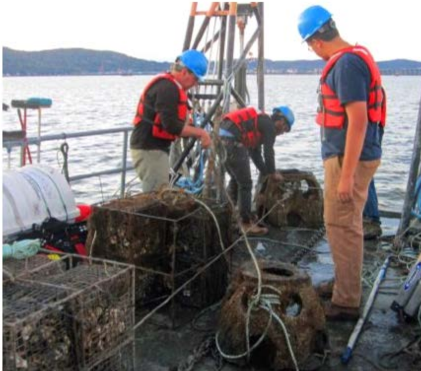
Figure 4. Hard substrates to be deployed in the Tappan Zee region of the Hudson River to promote the growth of oyster reef habitat include oyster shell-filled metal gabion cages (top left) and concrete Reef Balls (top right). Deployment of pilot substrates is shown at bottom.
