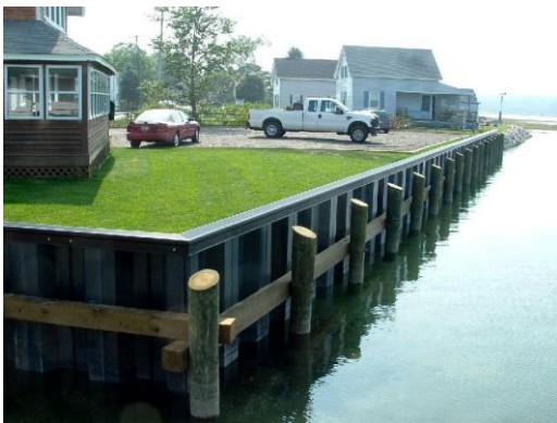
Hardened bulkhead shoreline in Scarborough, ME. Source: Maritime Construction and Engineering, LLC
