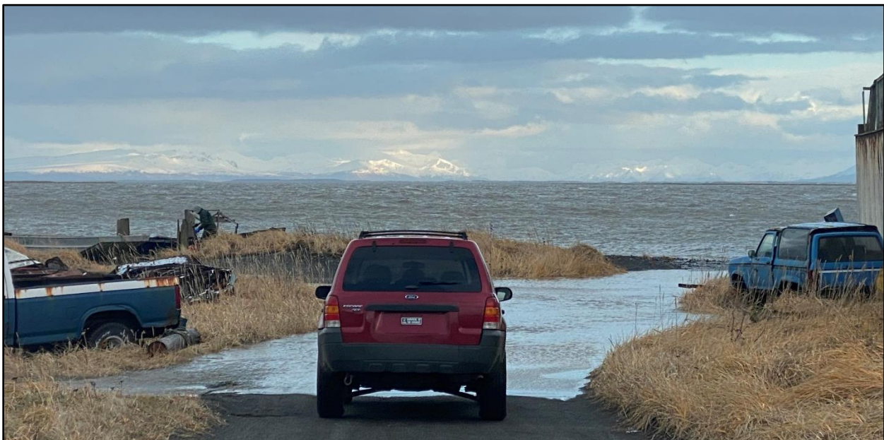
Figure 44. A flooded road near the retaining wall on the east side of the community . This stretch of coastline floods regularly during high storm-tides. Image provided by Angela Johnson, November 2020.
