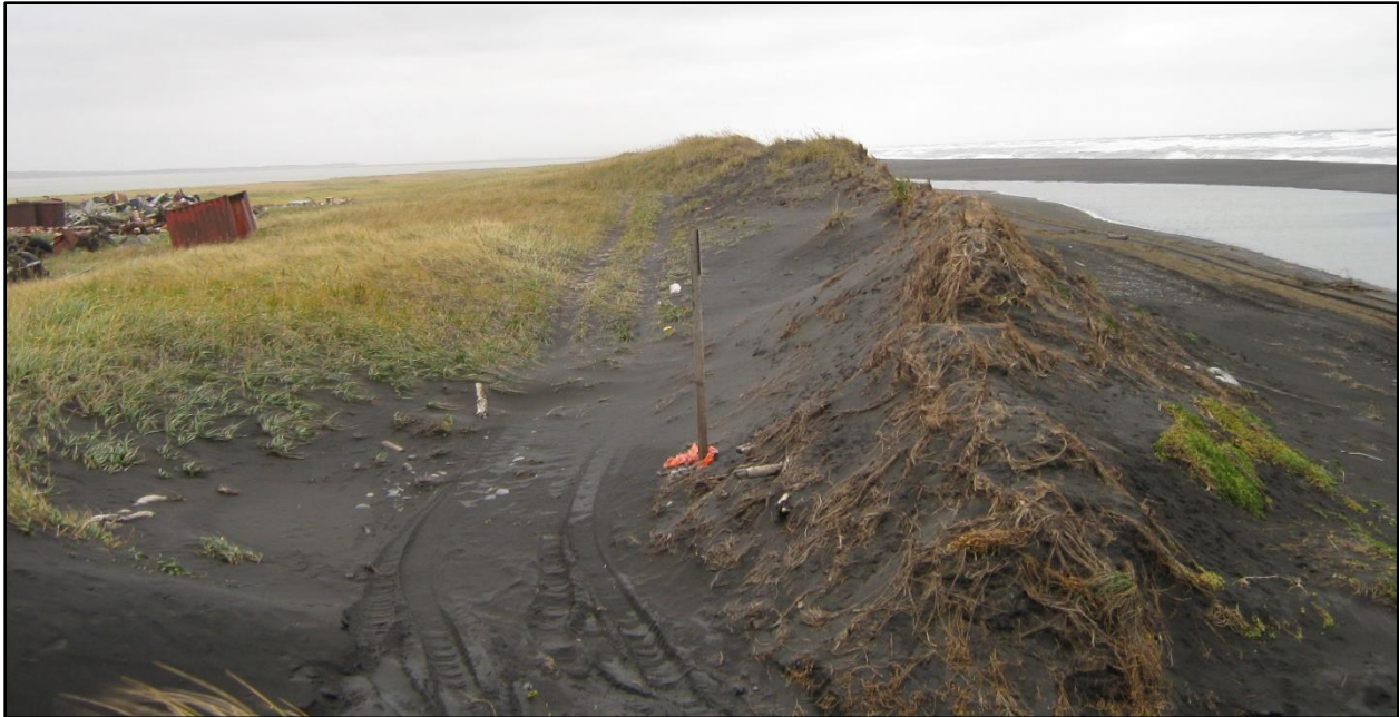
Figure 39. Photograph showing remnants of an overwash and flooding event at the access road from the beach to the solid waste disposal site, which can be seen to the left. October 2018.
