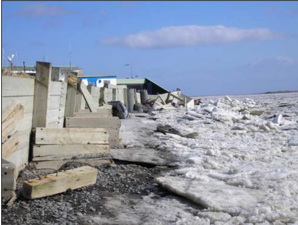
Figure 17. Bench ice along the Nelson Lagoon sea wall in 1995. Image Credit: HDR, 2011
