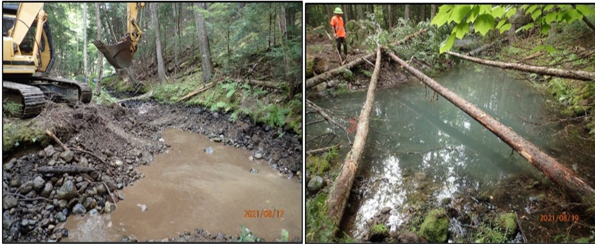
Figure 5.3.7. Groundwater Pool B2 during construction (left above) and after completion (right), Narraguagus River, Maine (2021). (credit: Chris Federico, Project SHARE)
