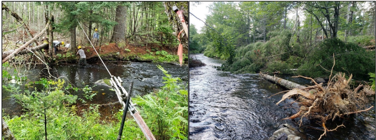
Figure 5.3.5. Preparing a tree for felling (left) and a completed wood jam (right) during a Griphoist wood addition, Narraguagus River, Maine (2021). (photo credit: Chris Federico, Project SHARE)
