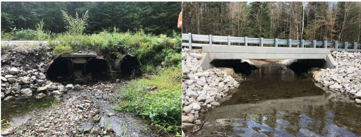
Figure 5.3.3. Cummings Brook crossing, before (left) and after (right) culvert replacement, Sandy River watershed, Maine 2021. (photo credit: Bill Bennett – USFWS-GOMCP)
