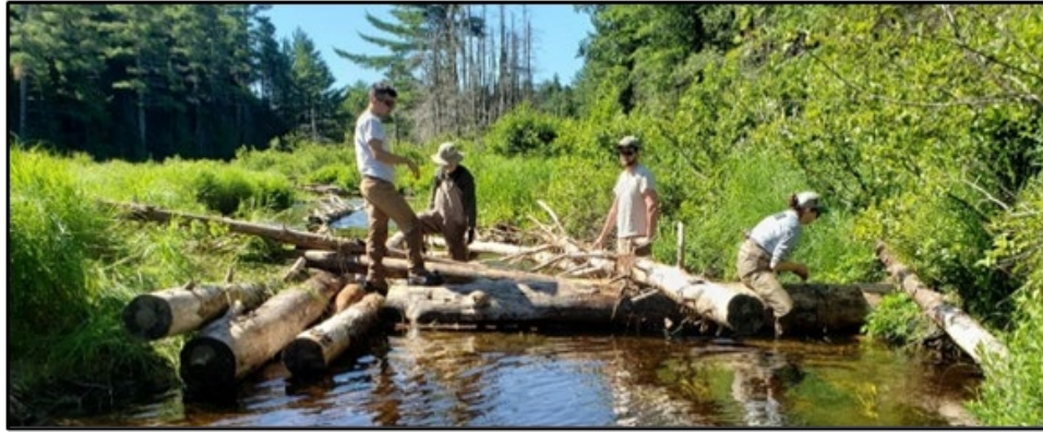
Figure 5.3.4. Constructed log jam with crew lashing the logs together, West Branch Brook, Maine (2021). (photo credit: Chris Federico, Project SHARE)
