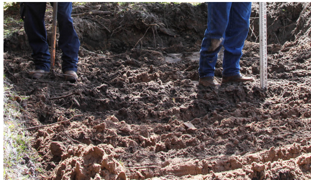
Raking the rain garden base
