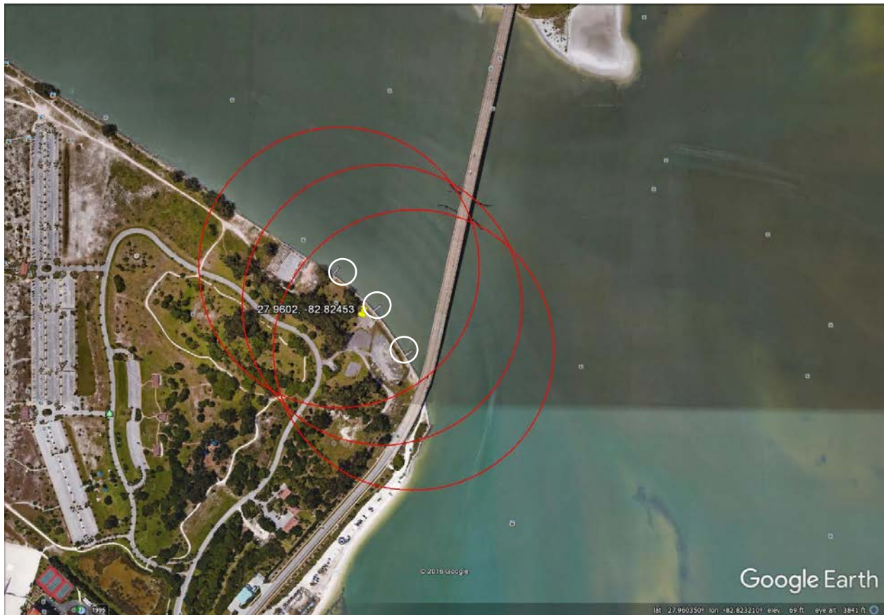
Figure 4. Image showing the action area for the Clearwater pier extensions – with an approximate noise impact radius of 705 ft extended outward from the site where behavioral effects to ESA-listed species may occur during pile driving during pier T-head construction (©2016 Google); white circles indicate the 3 existing piers.
