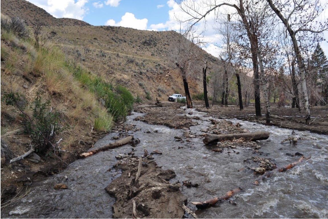
Figure A-7. The lower section of the obliterated road at Site #1. The road was located along the toe of the slope where the stream is now flowing (photograph taken on August 18, 2014).
