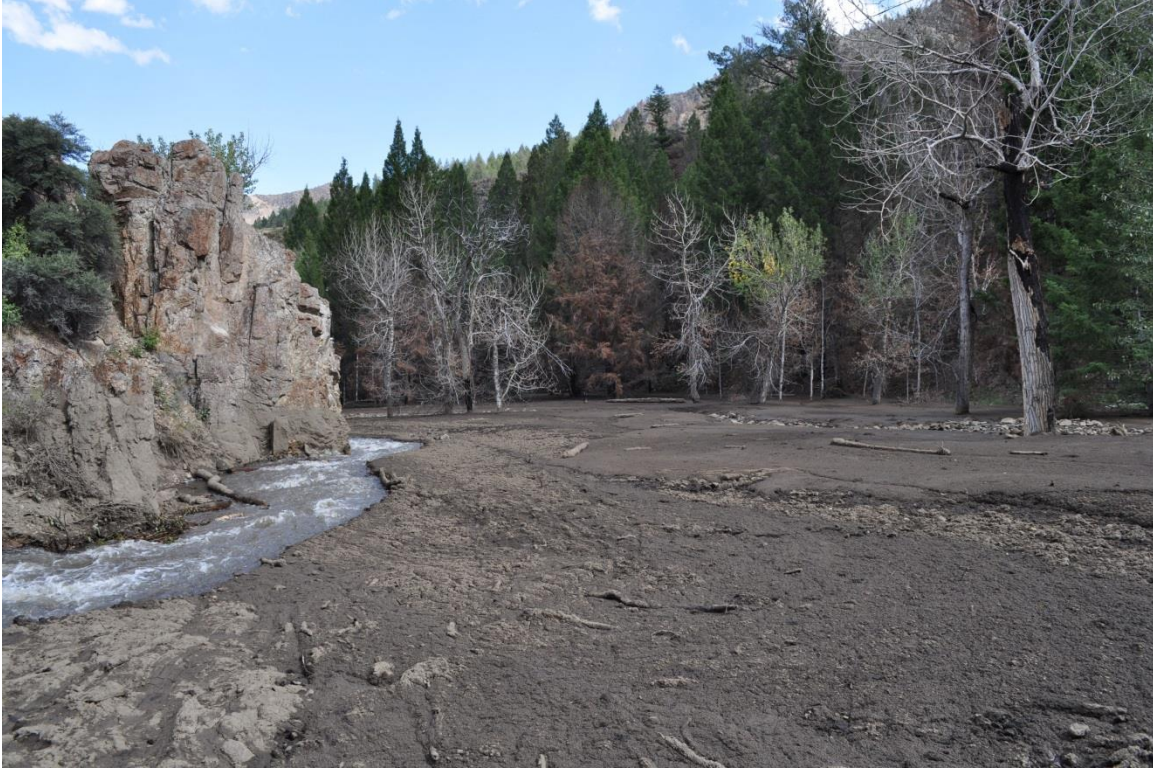
Figure A-5. The upper section of the obliterated road at Site #1. The road was located along the base of the small cliff where the stream is now flowing (photograph taken on August 18, 2014).
