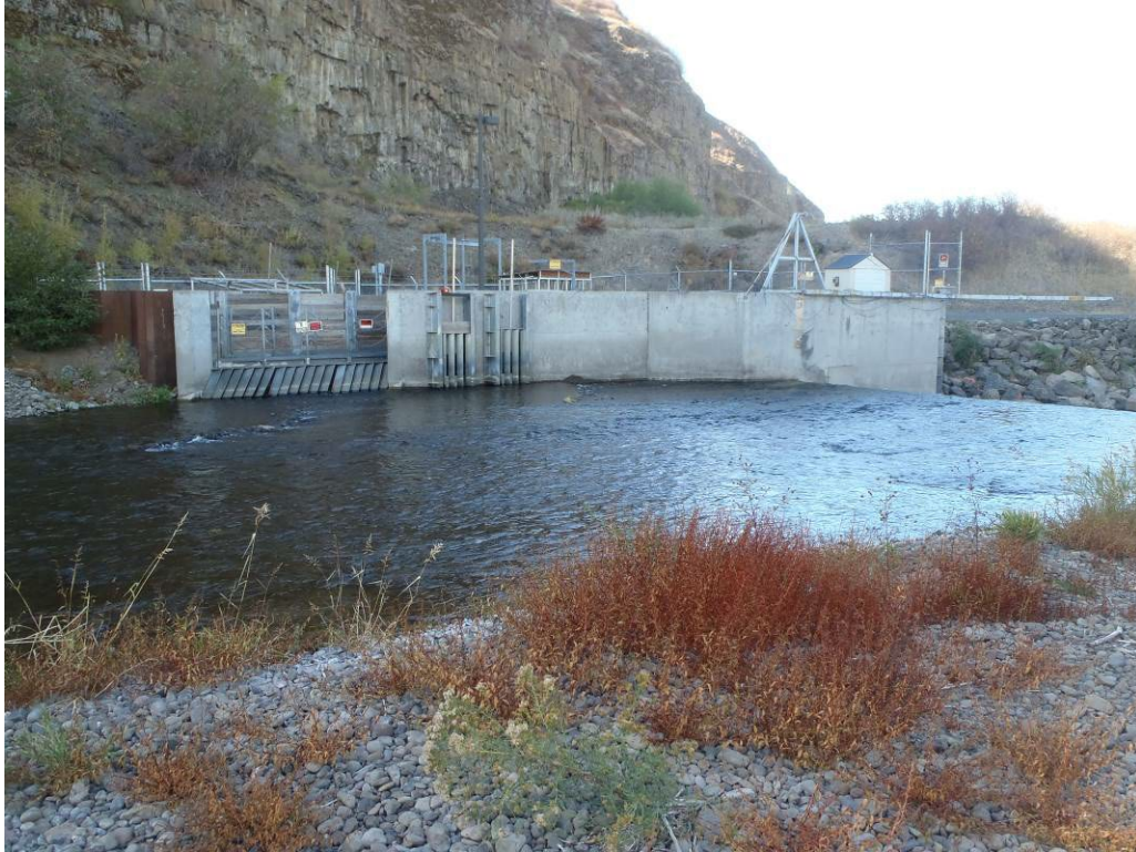
Photograph 3 (October 2021). Intake/Fish Ladder looking Southwest.
