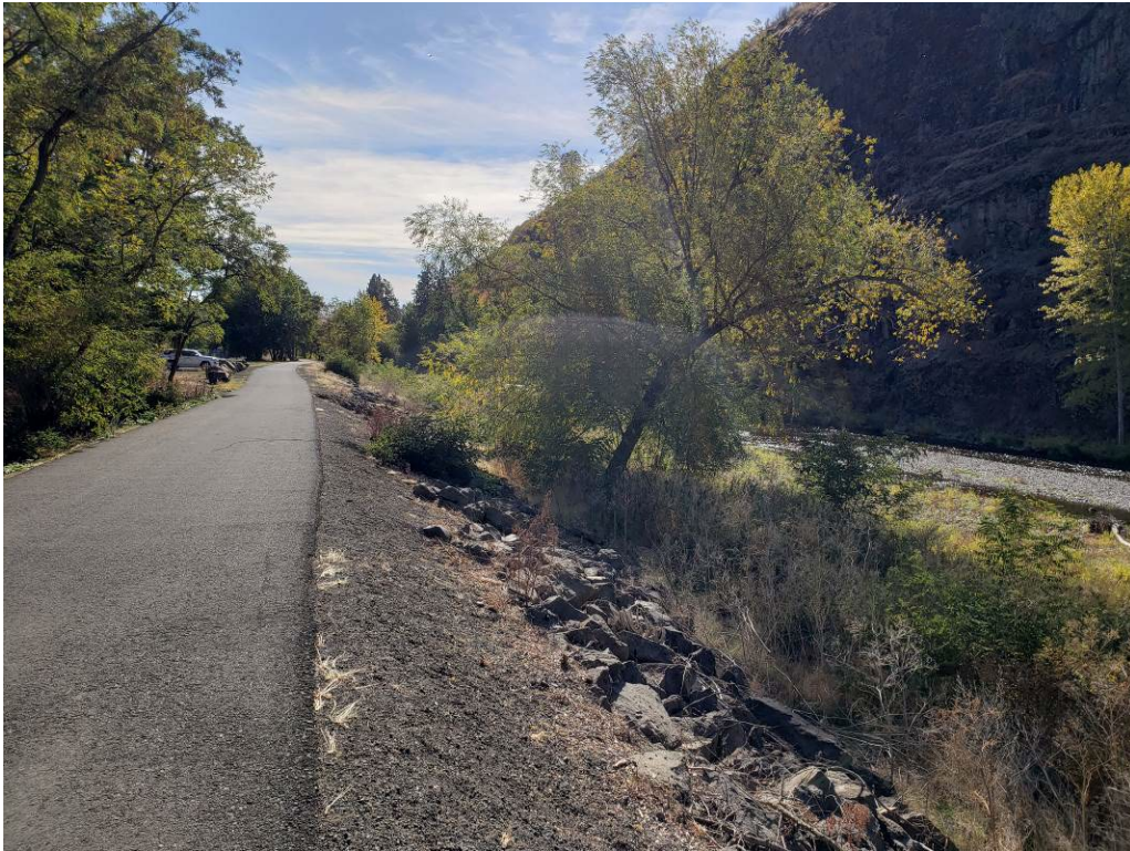
Photograph 9 (October 2021). USACE Levee adjacent to Touchet River looking Southeast.
