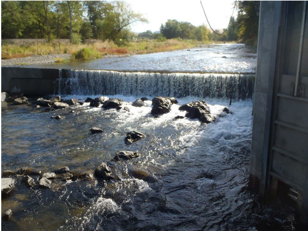
Photograph 5 (October 2021). New Obermeyer Weir Area looking Upstream.
