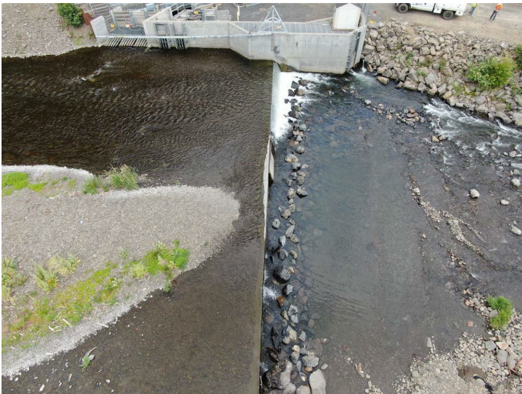
Photograph 2 (July 2021). Aerial View of Weir and 2021 Emergency Riprap Installation.
