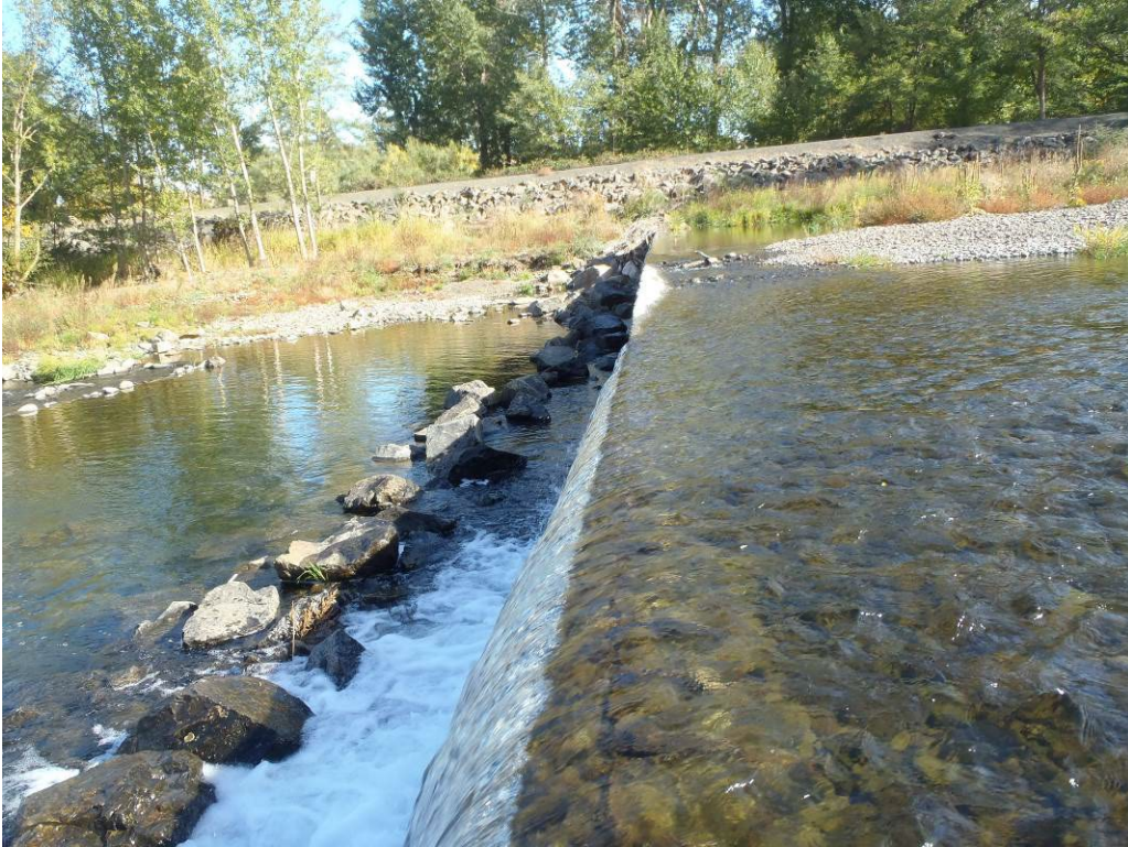
Photograph 7 (October 2021). Weir and Riprap looking Northeast.
