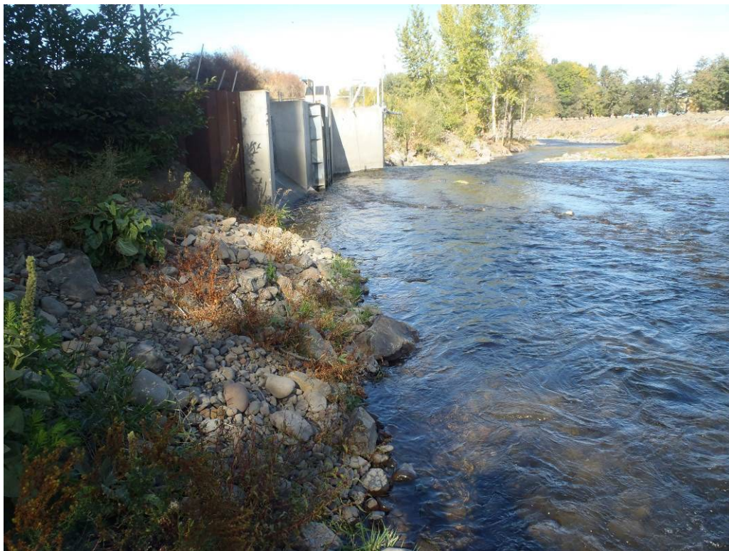
Photograph 4 (October 2021). Gravel Dredging Area Upstream of New Obermeyer Weir looking Downstream.
