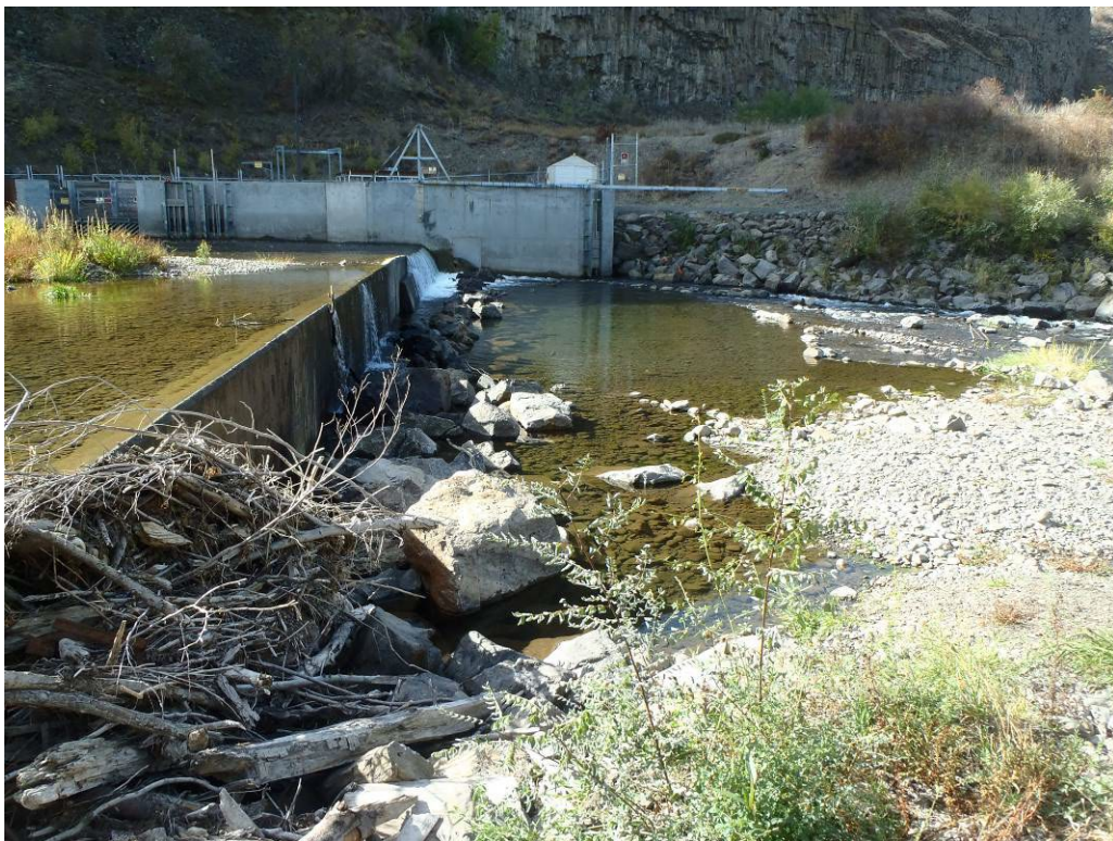
Photograph 6 (October 2021). Weir and Riprap looking Southwest.
