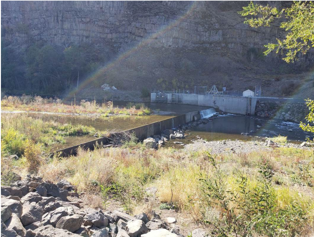
Photograph 1 (October 2021). Weir looking Southwest from USACE Levee.
