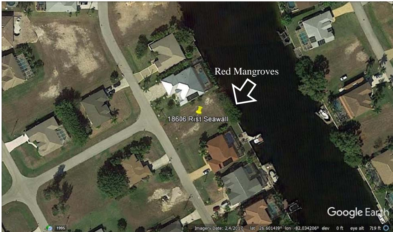
Figure 1. Image showing Gary Rist project location in a residential canal in Cape Coral, indicated by white rectangle, 40 lin ft of red mangroves indicated by white arrow (©2017 Google)
