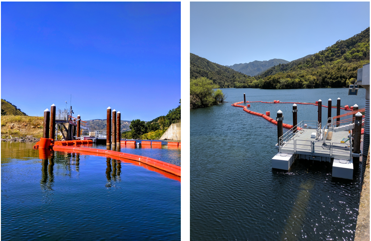
Figure SA1: Views of both the entrance and exit to the floating weir collector (FWC) located in the Los Padres reservoir. The entrance to the FWC, on left, and the exit pipe, on right.
