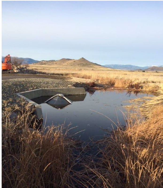
Figure 3. Shasta Valley Wildlife Area Diversion with cone screen over intake pipe (CDFW 2016).
