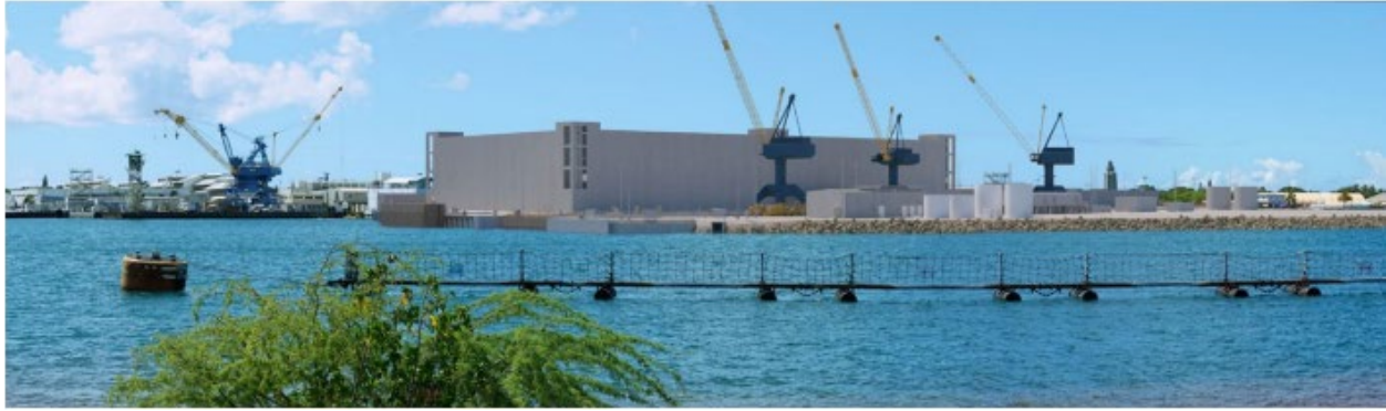
Figure 4. Visual simulation of WPF located adjacent to the dry dock (source: Navy Factsheet: https://www.pearlharbordrydockeis.org/api/files/6bb1ae0f-37a4-439e-9419-d498f7bdad3f ).
