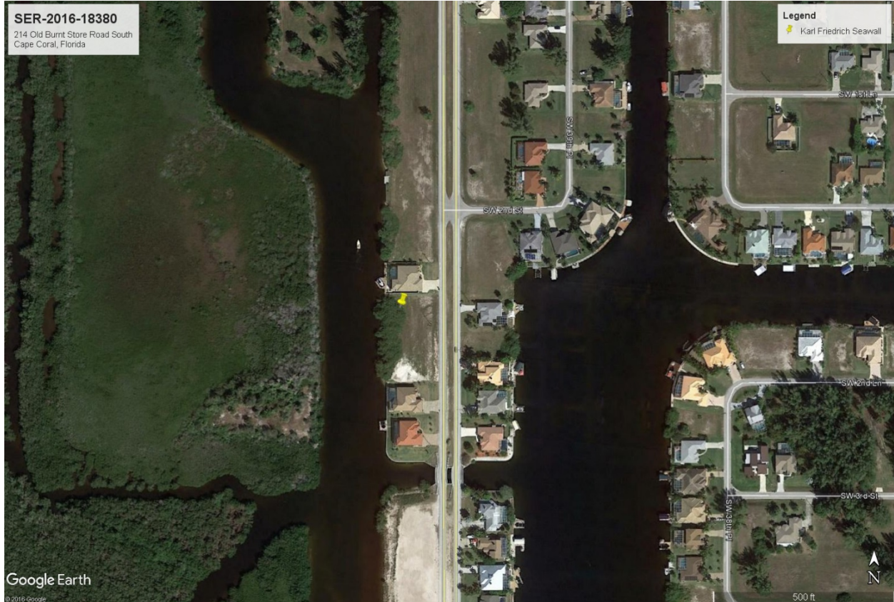
Figure 1. Image showing Karl Friedrich Seawall project site location and action area in the North Spreader Waterway in Cape Coral, Lee County, Florida (©2016 Google).
