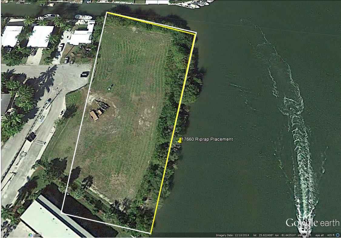
Figure 1. Image showing James Inglis shoreline stabilization (riprap) project location adjacent to Coon Key Pass in Goodland, Florida, (©2016 Google), shoreline where riprap will be placed outlined in yellow.
