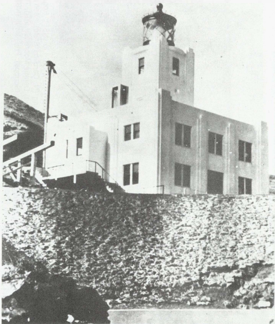
Scotch Cap Light Station, destroyed by Tsunami of 1946, killing all five occupants. Built in 1940 of concrete to replace a wooden structure built in 1903, it stood 60 feet high and 92 feet above water level. (Credit: U.S. Coast Guard.)
