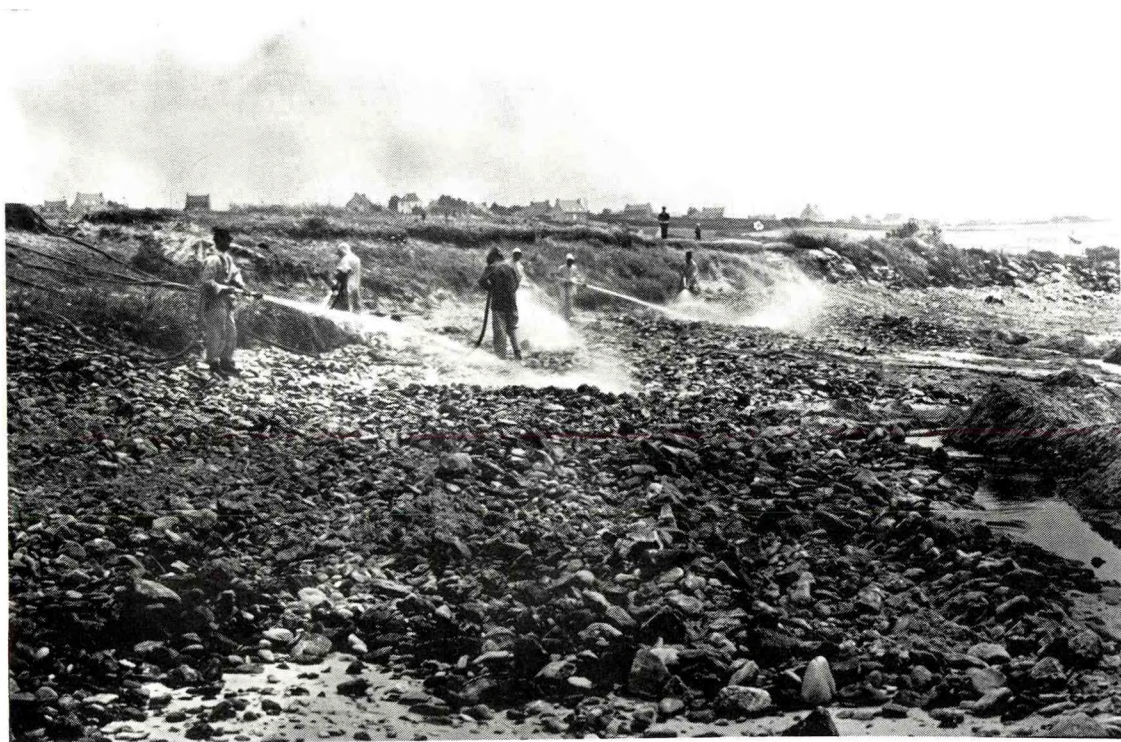
Figure 8. The clean-up of the oiled cobble area at station F-39 as observed on 18 July. Notice the trench at the right which was dug to capture oily runoff which would later be pumped out.
