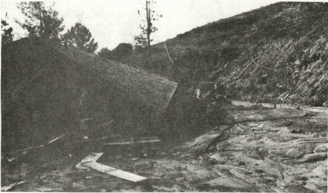
Figure 1.2--This home is one of many in the Los Angeles area severely damaged by mudslides. It was impacted by many tons of mud from the hillside in the background. This was the second time in 2 years that the homeowner lost his house to mudslides.
