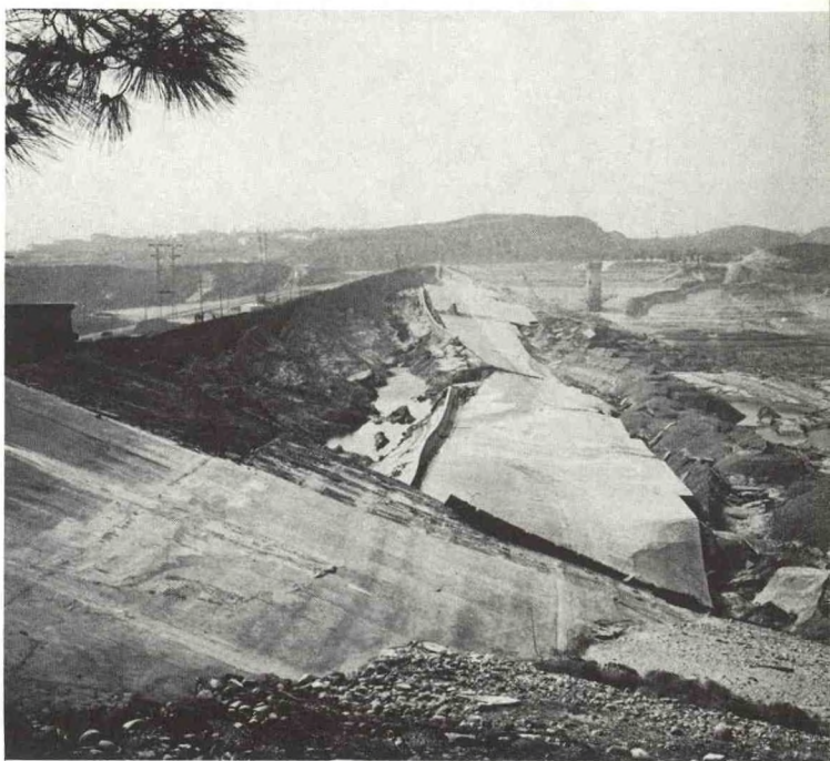
View showing failure of Lower San Fernando Dam and floor of Lower Van Norman Lake after drainage of water.
