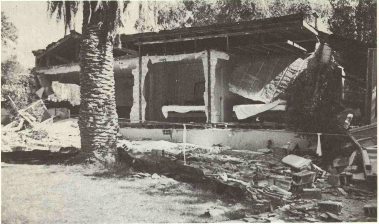
Exterior walls stripped from residence.
