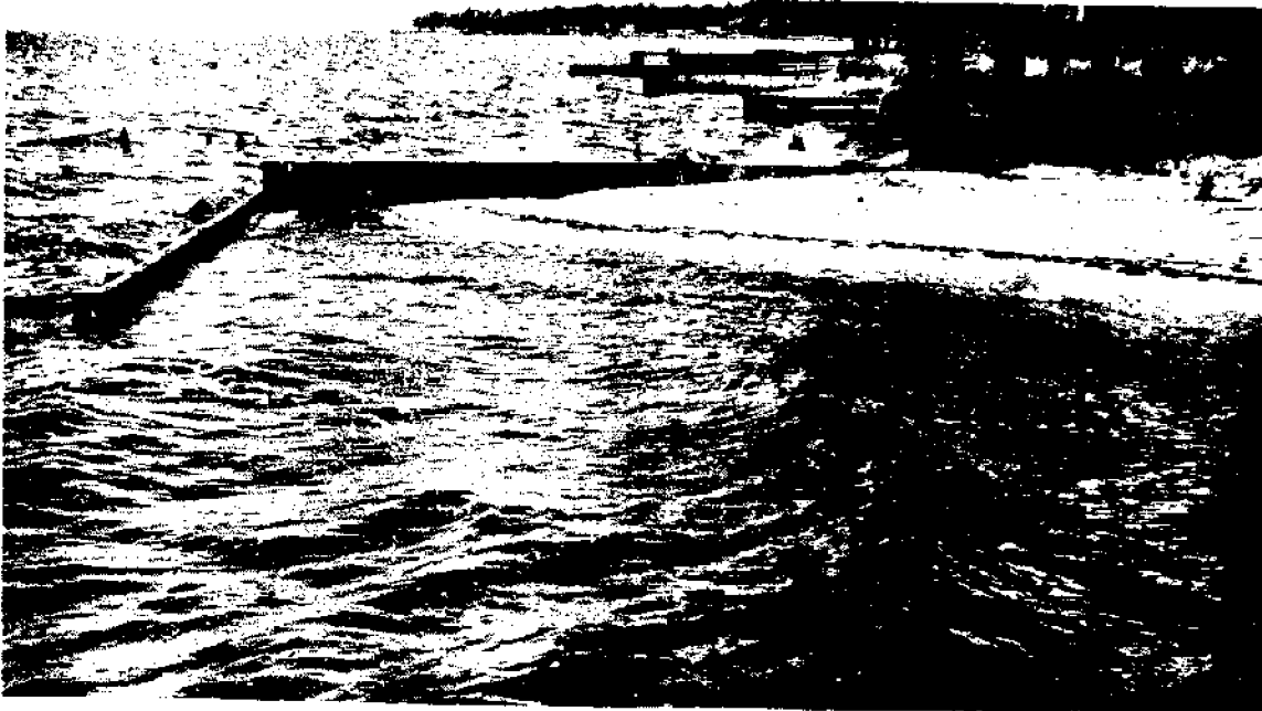
Figure 39. Groins constructed perpendicular to the shoreline are often effective in trapping sand transported along the beach. Groins become progressively less effective as new ones are added because all groins must compete for the limited amount of sand being moved by nearshore currents. In a very real sense the decision of one landowner to install groins will affect the rate of erosion of adjacent properties. Groin effectiveness is dependent upon continual input of fresh supplies of sediment eroded from the shoreline. Bulkheading eliminates the source of sediments needed to make groins effective. Photo taken along north shore of the Pamlico River, Beaufort County, N. C.
