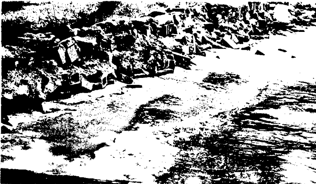
Figure 37. Bulkheads of original design such as the one illustrated here are moderately successful if constantly maintained with back fill and restacking of blocks. Many waterfront owners consider such structures to be unsightly. Certainly they are a real nuisance to maintain.
