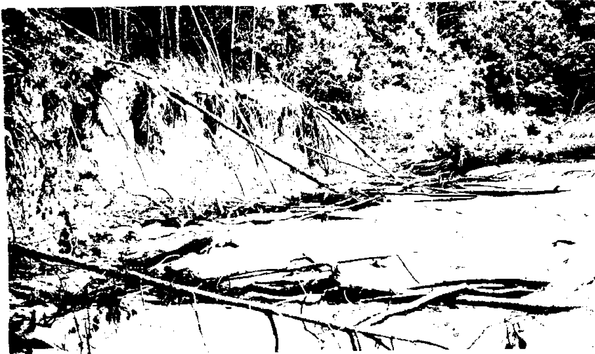
Figure 13. Rapid erosion occurs wherever the low bank contains a high sand content. Concave banks undercut the trees and they are blown over into the water by strong offshore winds. Such wind-thrown timber may act as a natural groin with the sediments captured tending to retard further erosion. Photo taken near Greenfield Plantation, Chowan County, N. C.
