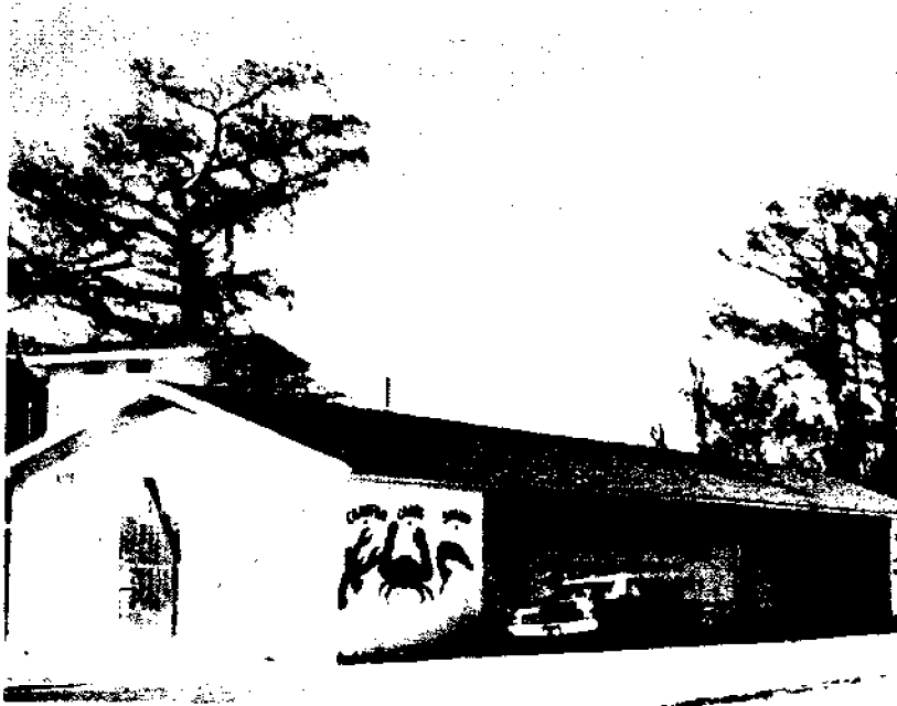
Figure 25. A processing plant near Pierre Part.
