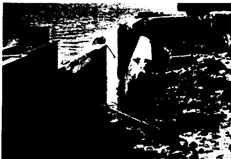
Fig. 23. Advanced stage of loss of supporting backfill
