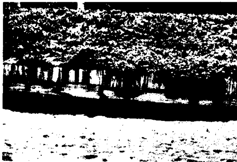
Fig. 2. A wooden bulkhead installed in 1928, still in good condition after 46 years of service, just south of Boynton Inlet in Palm Beach
