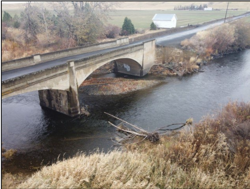
Photograph 1- Existing Dell Sharpe Bridge (facing north)
