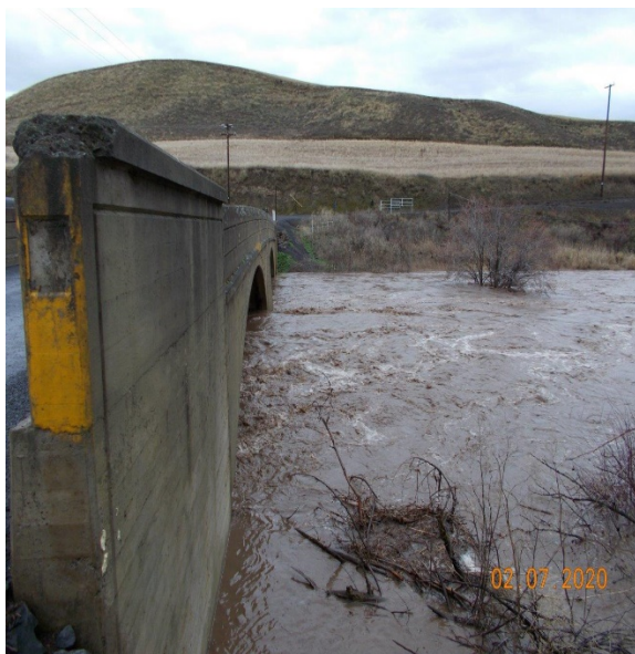
Photo 7. +100 year flood level at bridge
