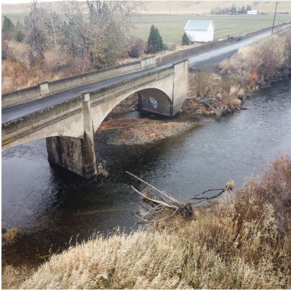
Photo 1. Upstream of Bridge facing north
