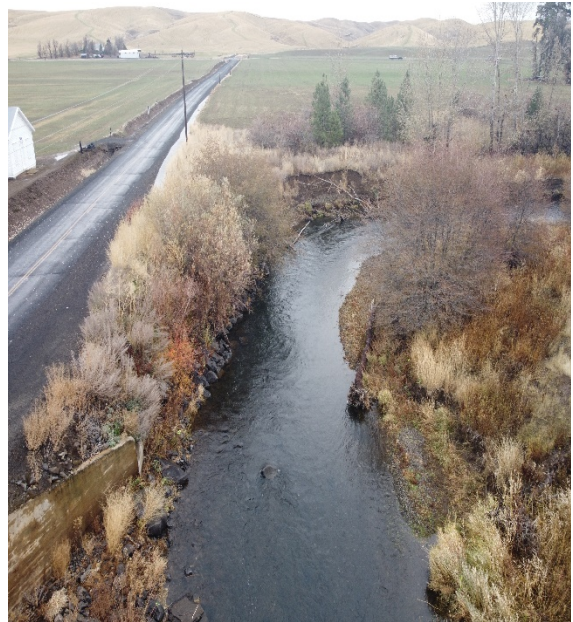
Photo 4. Meander at bridge (facing north)
