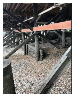
Figure 19. Removal Credits for Non-Functional Shoreline Armoring that is not in good condition. Removal credits do not apply for horizontal pile stabilizer as there is no functioning bulkhead effect (like sediment retention behind the bulkhead or elimination of water exchange).
