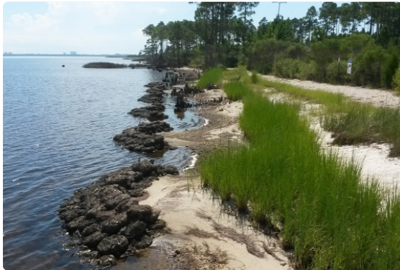
Living Shoreline constructed in Panama City, Florida using plants and oyster shell. Photo: Florida Living Shorelines
