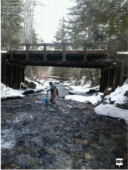
Figure 56. North Fork Taneum bridge showing existing abutments, riprap, and bankfull widths.
