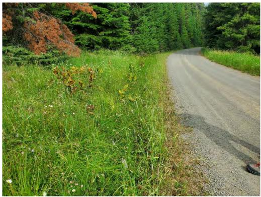
Figure 61. Effective ditch on upslope side of existing system gravel road. A temp road is proposed on the upslope side of the road and an intermittent stream is on the downslope side.
