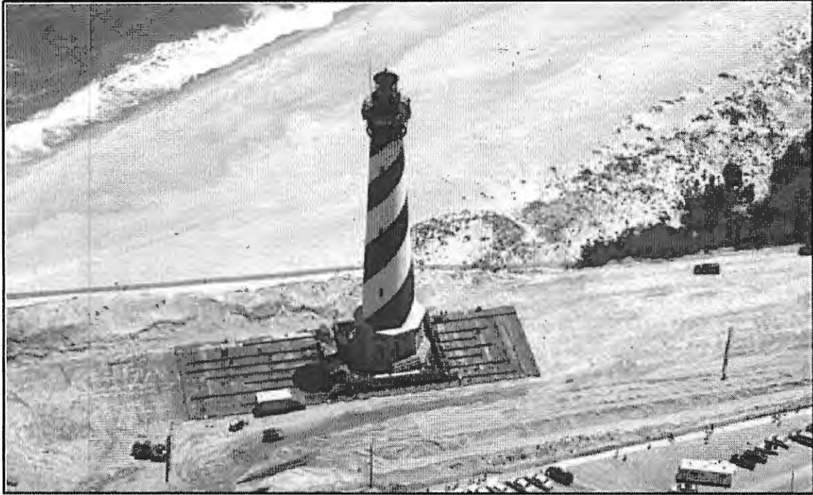
Figure 1-34. Cape Hatteras Lighthouse is on its slow and deliberate move towards the new inland relocation site. Photo is by the N.C. Department of Transportation.
