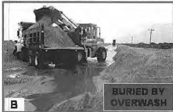
Figure 2-12. N.C. Hwy. 12 “going-to-sea” as the storm tide washes over the road during a typical nor’easter. In some storms the highway is just buried in overwash sand that is cleared off the road and put back into a barrier-dune ridge. Other storms physically destroy the road as it finds itself in the surf zone. Photograph A is by O.H. Pilkey, B is by S. Riggs, and C is by Cape Hatteras National Seashore personnel.
