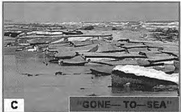
Figure 2-12. N.C. Hwy. 12 “going-to-sea” as the storm tide washes over the road during a typical nor’easter. In some storms the highway is just buried in overwash sand that is cleared off the road and put back into a barrier-dune ridge. Other storms physically destroy the road as it finds itself in the surf zone. Photograph A is by O.H. Pilkey, B is by S. Riggs, and C is by Cape Hatteras National Seashore personnel.
