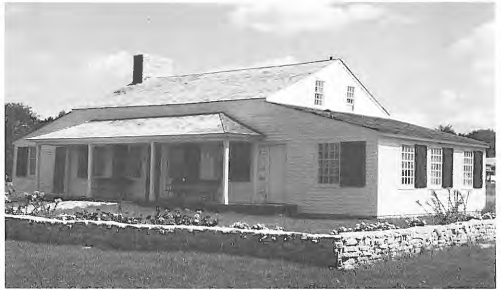
Roi-Portier-Tank Cottage. Photo by Margaret Bogue.
