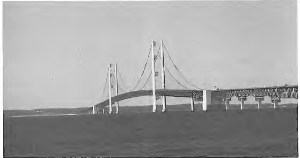
Mackinac Bridge spanning the Straits viewed from Fort Michilimackinac. Photo by Allan Bogue.
