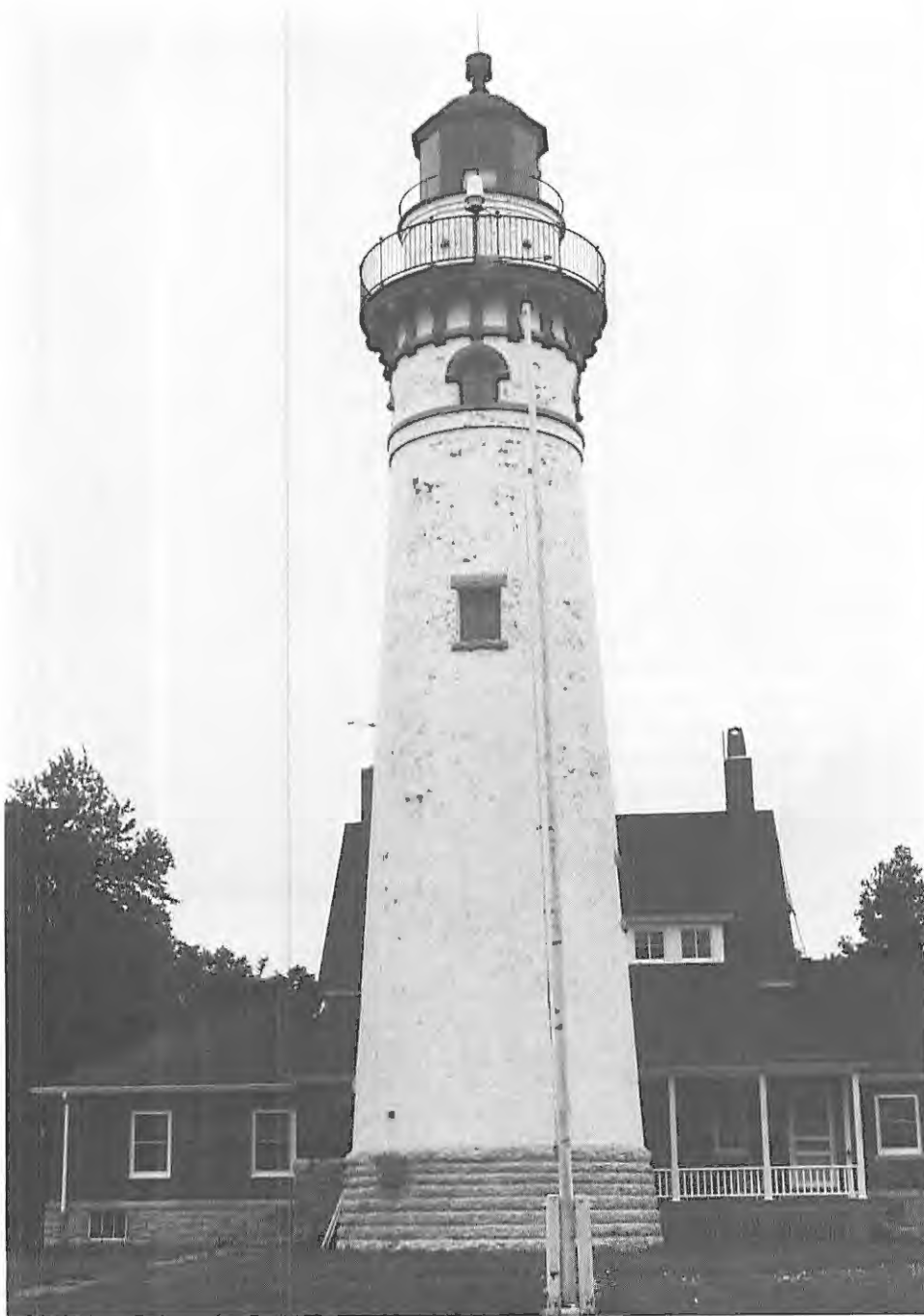
Seul Choix Point Lighthouse is one of a number built on the Great Lakes and elsewhere by the federal government in the late nineteenth century using the same architectural design. Note the Italianate bracketry and curved window design at the upper level. Photo by Margaret Bogue.
