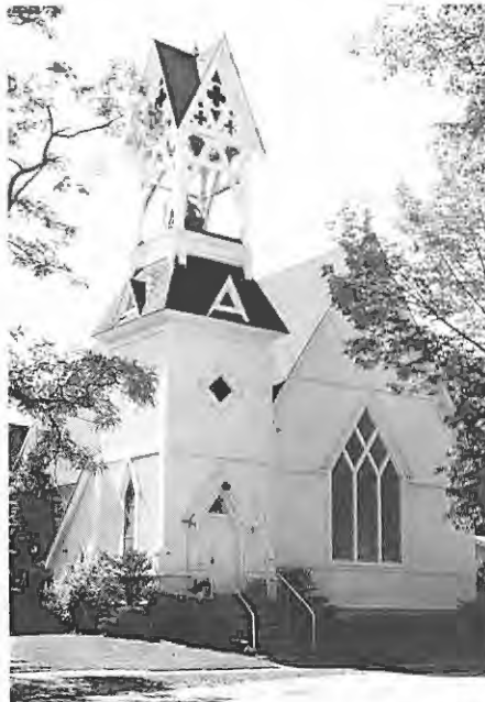
St. Paul's Episcopal Church is probably the finest building architecturally in Elk Rapids. Photo by Margaret Bogue.
