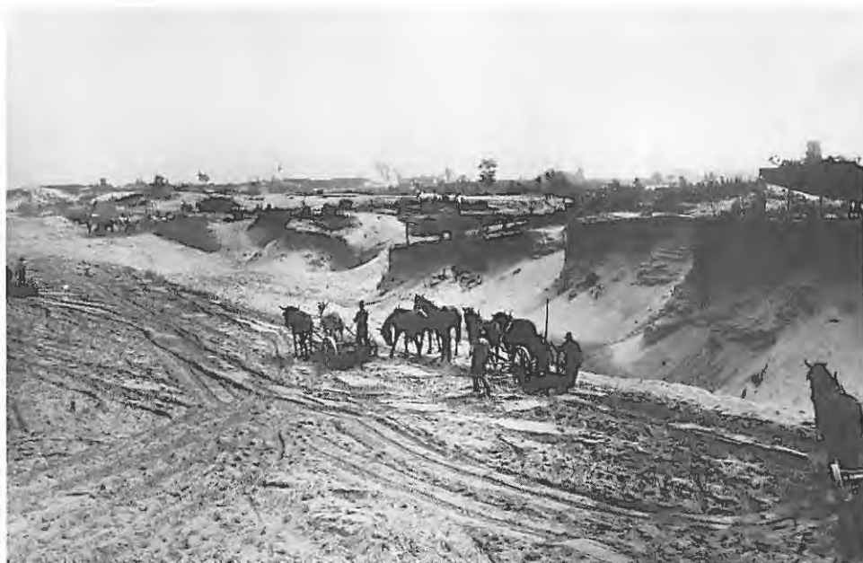
Grading and leveling in preparation for construction of the U.S. Steel plant. Courtesy U.S. Steel Corporation.
