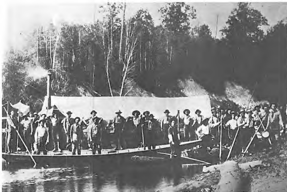
Batteau crew whose job it was to keep the logs moving on the river drives and the wanigan, boat that carried food, cook, cook's helpers, and tents for the journey from the pineries to the mills. Muskegon River, 1888. From the Collections of the Michigan State Archives, Department of State. 07951
