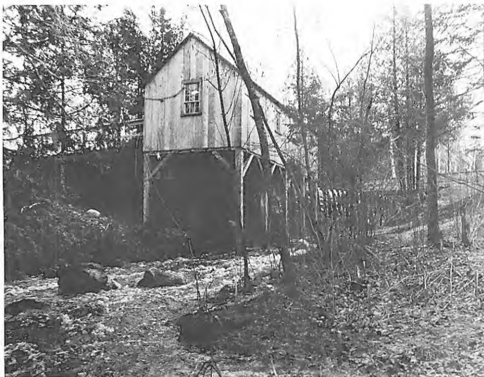
The Mill and mill stream. Courtesy Michigan Department of Natural Resources.
