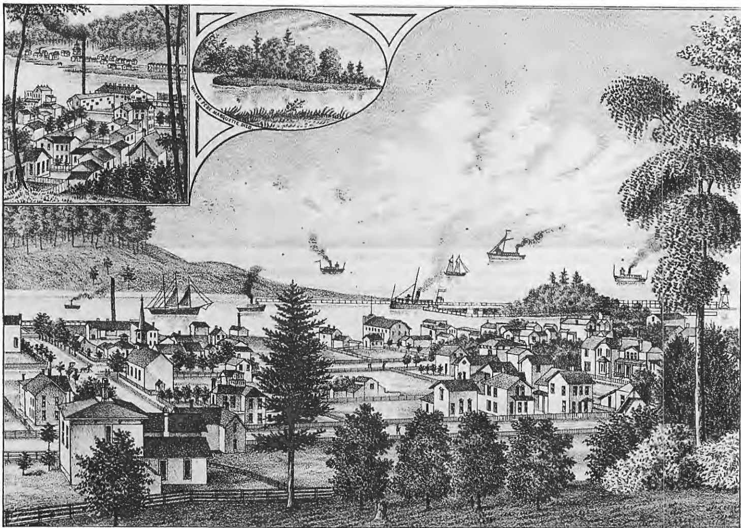
The Frankfort Harbor about 1875 is the central focus. Note as well the upper left inset of South Frankfort, later renamed Elberta. The oval inset stakes Frankfort's claim to being the place where Jacques Marquette died. The Ludington versus Frankfort controversy still continues. Courtesy State Historical Society of Wisconsin. WHi(X3)40553
