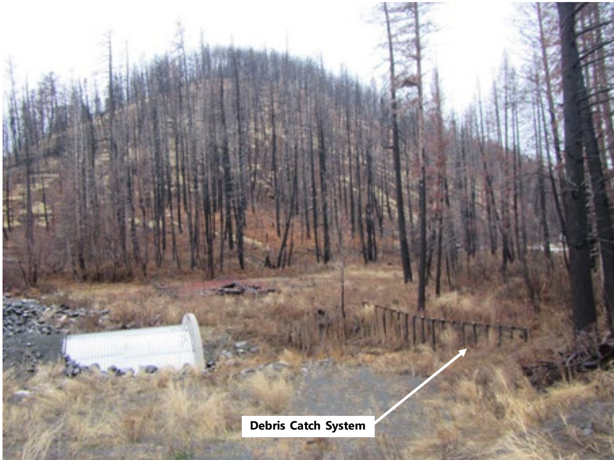
Figure 20 Debris Catch System Installed Upstream of a Culvert on Vance Creek, Oregon Following a Wildfire
