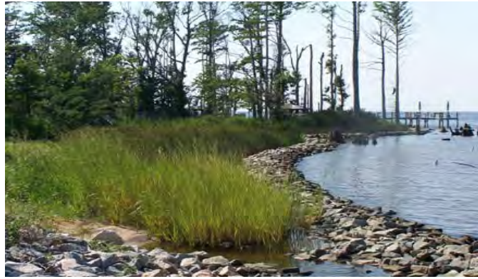
Marsh Sill (Photo: N.C. Division of Coastal Management)
