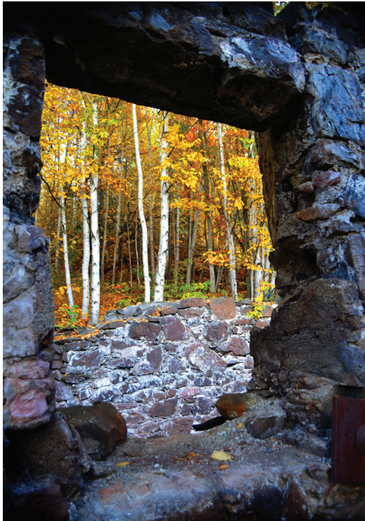
Ruins of Quincy powerhouse. Photograph by Todd Marsee, Michigan Sea Grant, 2012.
