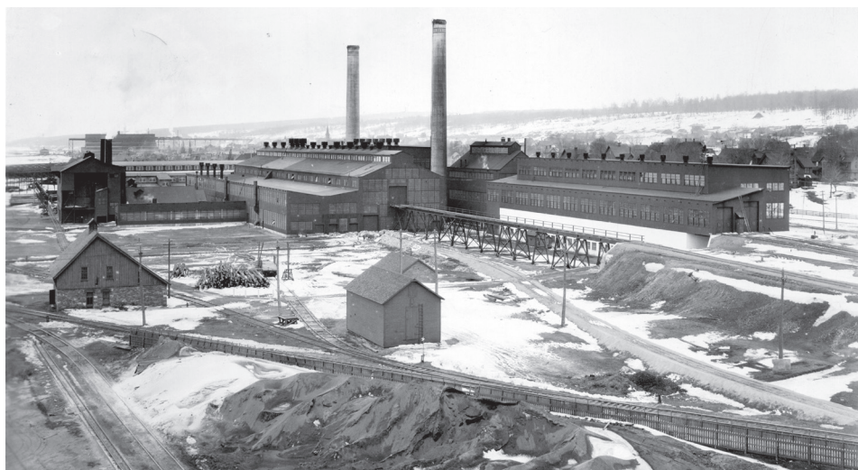
Photograph of C&H smelter and concentrate storage building in Hubbell, MI about 1950. Photo provided by the Michigan Technological University Archives and Copper Country Historical Collections.
