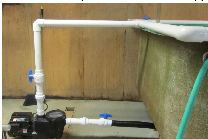
FIGURE 4: PVC CONNECTIONS GOING FROM TANK DRAIN TO PUMP INLET, THEN PUMP OUTLET TO PVC RING
