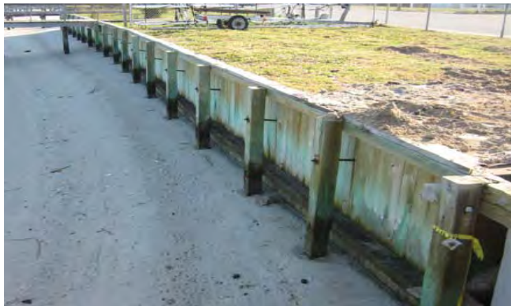
Bulkhead (Photo: N.C. Division of Coastal Management)
