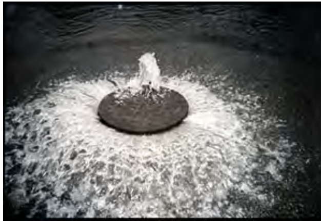
SSOs may allow wastewater to flow onto public areas, such as streets. 285
