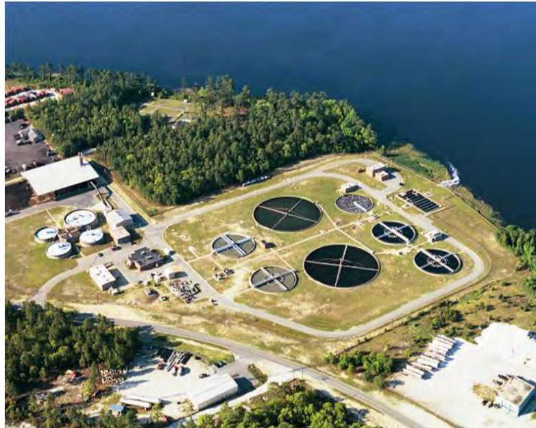
McKean-Maffit (Southside) Wastewater Treatment Plant in Wilmington 329
