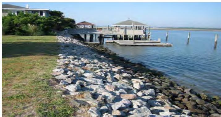
Revetment (Photo: N.C. Division of Coastal Management)
