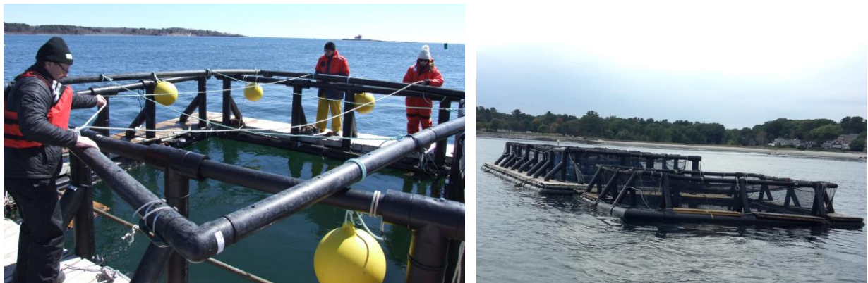
Figure 20: (left) The frame lifted on top of the IMTA raft. (right) The IMTA raft, located next to the Project SOAK frame system at the site.
