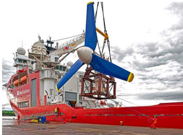
Figure 9: Atlantis Resources Corporation tidal turbine deployment in Orkney [12].
