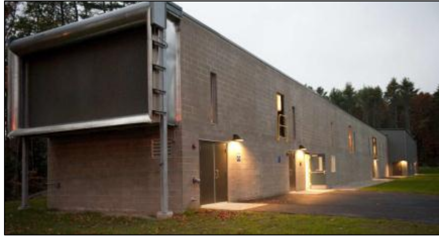
Figure 2: The UNH Flow Physics Facility, with test section dimensions W 6.0 m x H 2.7 m x L 72 m.
