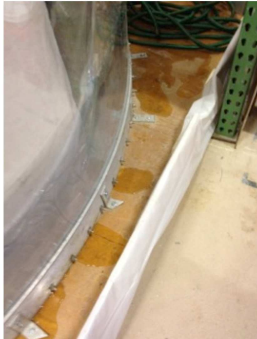
Figure 16: Leaks due to sliced hole in liner
