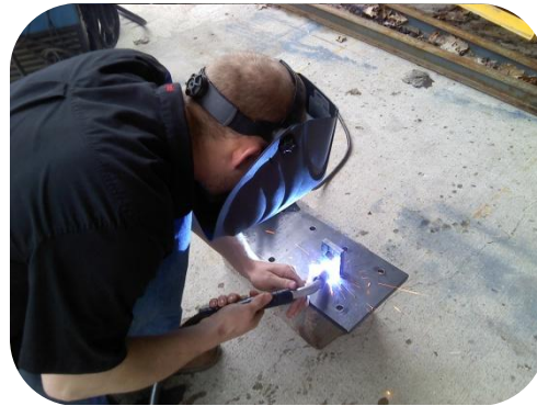
Figure 6.4: Welding of mounting bracket
