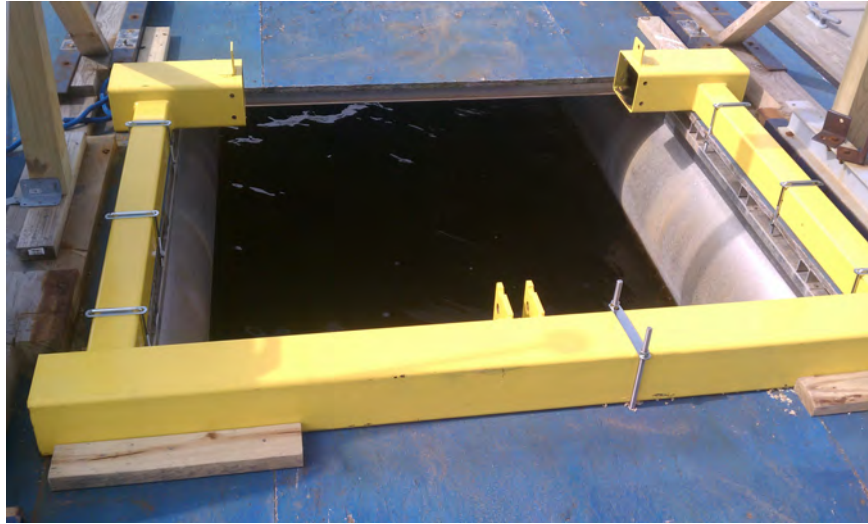
Figure 28: Completed top frame assembly mounted on the barge
