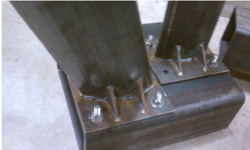
Figure 27: Plate and Gussets attached to the airfoil
