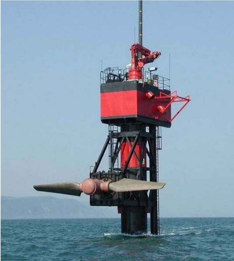
Figure 3: SeaGen prototype in Ireland, Predecessor to First Commercial Tidal Stream Generator
